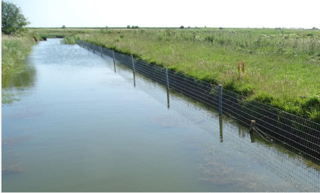
Fig. 3. A typical underwater/in-ditch fence, in this case with recycled plastic fence posts at Road's Farm, Frampton Marsh. This is part of a mixed fence that also includes a section of barrier fence that protects 52 ha of freshwater and brackish scrapes and other wetland habitat. The outside of the fenced area is to the left. Photo by Malcolm Ausden.
