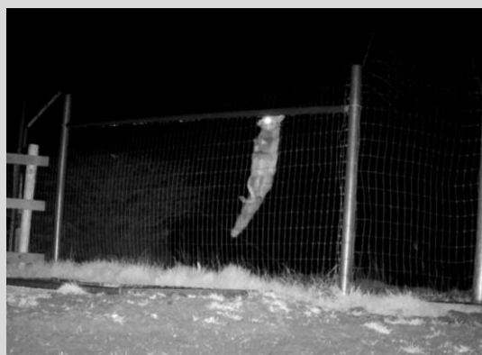
A Fox scaling the mesh of a 1.8 m high barrier fence before deciding it cannot get over its angled mesh top and jumping back down to the ground
