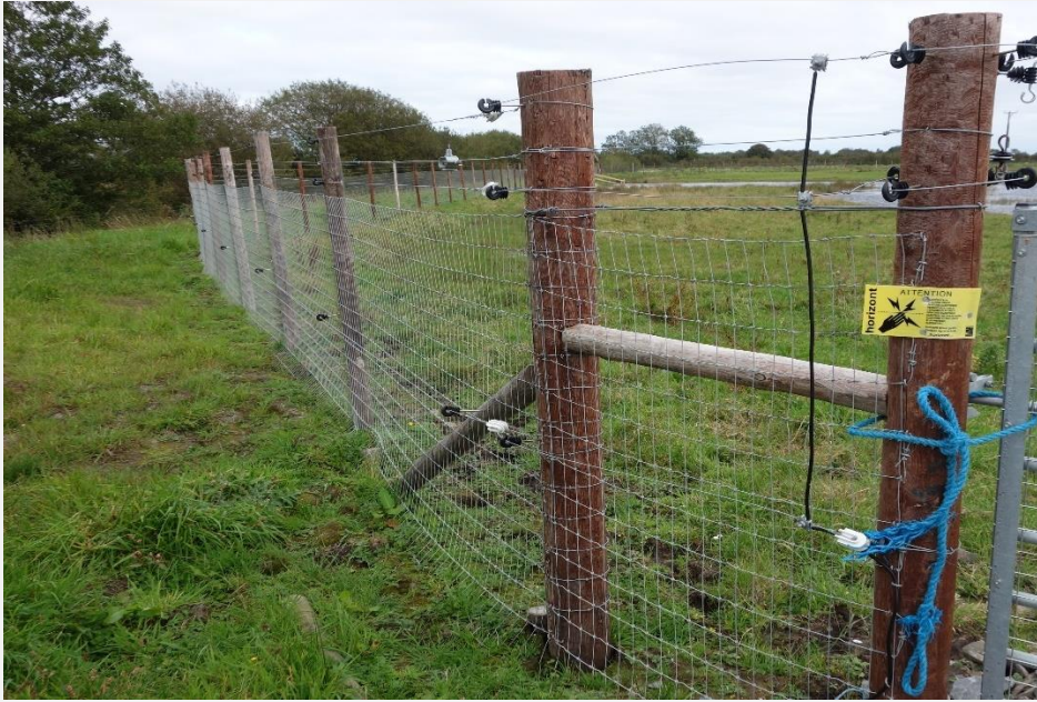
Fig. 1. A typical combination fence with wooden fence posts at Campfield Marsh. This has two live wires above the mesh with an earth wire between them, and one live wire offset lower down on the outer side of the mesh. The outside of the fenced area is to the left. Photo by Gavin Thomas.
