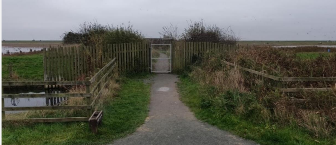
Fig. 26. (a) A pedestrian gate through an above-ground section of barrier fence that is connected to underwater fencing either side of it at Frampton Marsh. The upright wooden posts have been designed to prevent Foxes from climbing over them, but also to be more aesthetically pleasing than a typical metal barrier fence. They consist of 1.8 m high, half round, smooth pine posts with a floppy mesh top. The gate (b) is self-closing and comprises galvanised 1.2 m x 1.8 m frames with one inch weldmesh and an outwardly-angled mesh top. Photos by Toby Collett.
