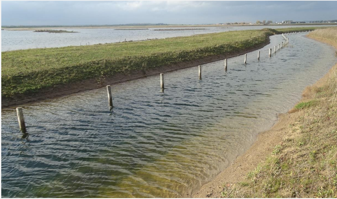
Fig. 29. A section of underwater fencing with chestnut posts in a specially-constructed ditch on Wallasea Island, with levels designed so that the top of the fence is below ground level and thereby invisible as you look across the landscape. This is part of an underwater fence that has successfully protected an area comprising 86 ha of wet grassland and 17 ha of saline lagoons from Foxes and Badgers. The outside of the fence is to the right. Photo by Malcolm Ausden.
