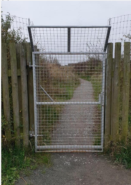
Fig. 26. (a) A pedestrian gate through an above-ground section of barrier fence that is connected to underwater fencing either side of it at Frampton Marsh. The upright wooden posts have been designed to prevent Foxes from climbing over them, but also to be more aesthetically pleasing than a typical metal barrier fence. They consist of 1.8 m high, half round, smooth pine posts with a floppy mesh top. The gate (b) is self-closing and comprises galvanised 1.2 m x 1.8 m frames with one inch weldmesh and an outwardly-angled mesh top. Photos by Toby Collett.
