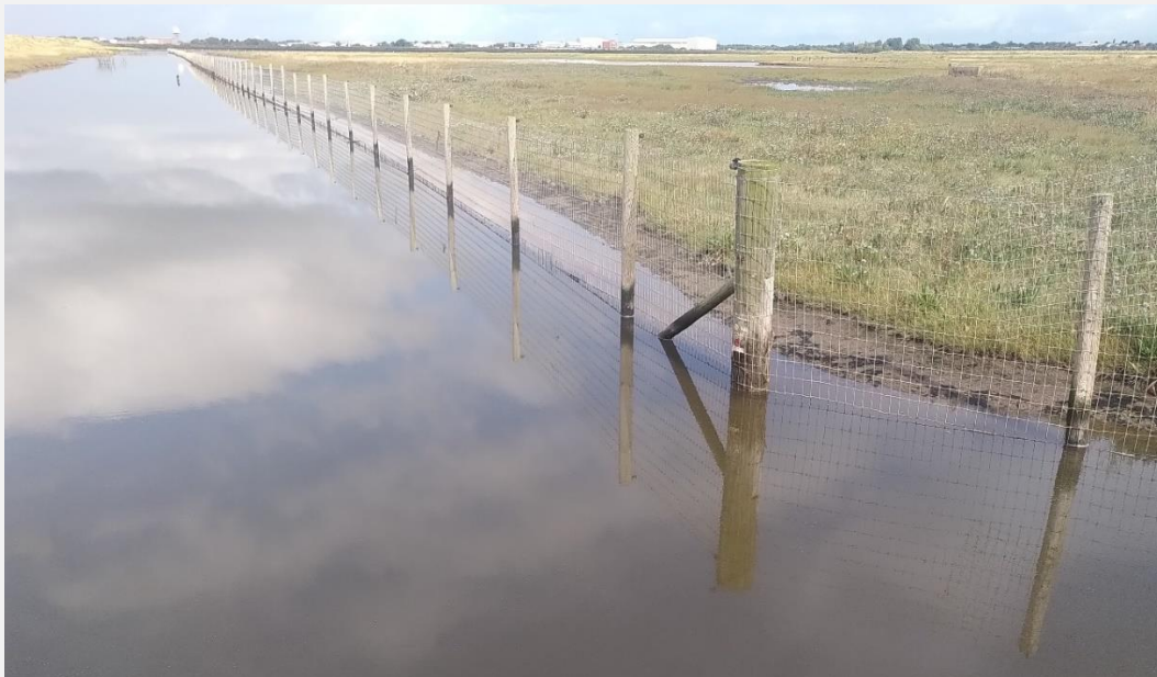
Fig. 19. Examples of combination fences installed along the edge of standing water. (a) A standard design combination fence installed along a ditch edge at Coveney Byall Fen. (b) A 140 cm high mesh fence with a single high tensile, galvanised, steel, live wire running along its top installed to enclose an area of saline lagoons and islands within an area of managed realignment at Hesketh Out Marsh East. Photos by Malcolm Ausden.
