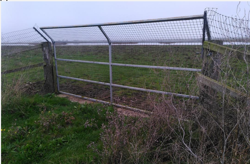
Fig. 25. Two slightly different variations in the design of gateway through sections of barrier fence (a) A modified Tornado 12' x 6' galvanised deer gate with an outwardly angled mesh top welded onto it, so that the top of the gate remains just below 2.0 m above ground level (see main text). The photo also shows the concrete plinth below the closed gate. This gate at Shorne Marshes East had only just been installed when the photo was taken, and the gaps between the gate and the fence either side were yet to be filled with mesh. (b) A mesh-covered gate with a rigid, outward facing-angled mesh top at Wallasea Island extending to 1.95 m above ground level. Photos by Malcolm Ausden.
