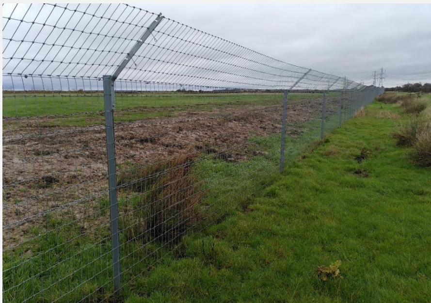
Fig. 2. A typical barrier fence with metal posts and a 'cranked' floppy mesh top at Shorne Marshes East. The outside of the fenced area is to the right. Photo by Malcolm Ausden.
