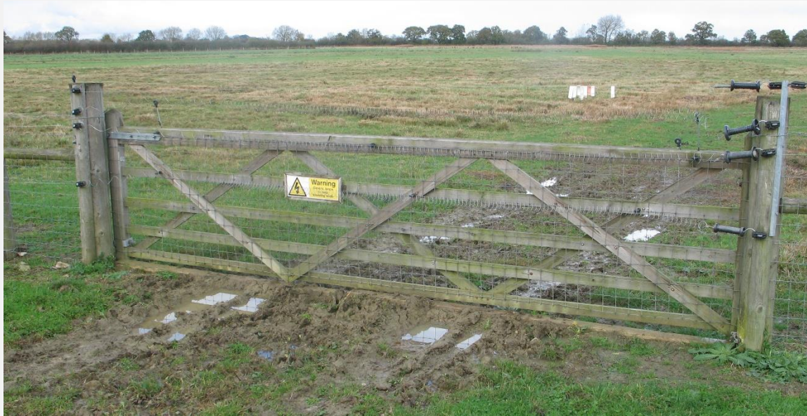
Fig. 20. A typical wooden gate in a combination fence at Otmoor, which has the three live wires of the rest of the fence running across it, two at the top and one halfway up the gate. These live wires can be detached and re-attached using the black bungees when the gate is opened and closed (see close-up to the left). Photos by David Wilding.
