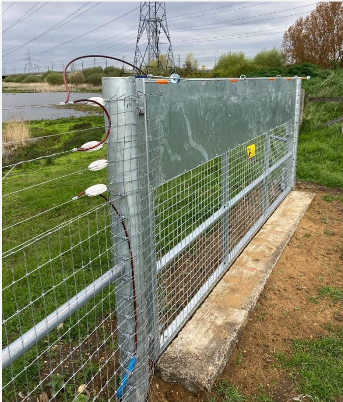
Fig. 22. An innovative design of gate through a combination fence at Rainham Marshes. The lower two thirds of the gate is covered by metal mesh on their outside, while the top third of the gate has a smooth metal panel across it. There is also a dead-end, live 'bar' running across the top of the gate to further deter animals from climbing/jumping over (see close-up below). The outside of the fence is to the right.
