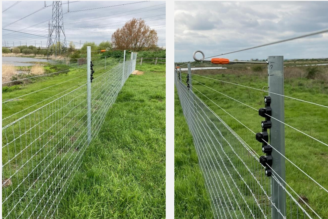
Fig. 18. Views from the outside of a combination fence at Rainham Marshes that has metal fence posts with four live, high tensile, galvanised, steel wires and an earth wire above its mesh, as shown in Fig. 16c. The black, Versalok insulators (see close-up on right hand photo) are stacked to reduce the gap between the live wires to 8 cm. Photos by Jamie Smith.
