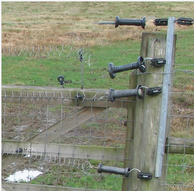
Fig. 20. A typical wooden gate in a combination fence at Otmoor, which has the three live wires of the rest of the fence running across it, two at the top and one halfway up the gate. These live wires can be detached and re-attached using the black bungees when the gate is opened and closed (see close-up to the left). Photos by David Wilding.
