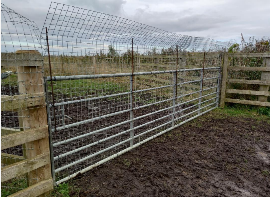
Fig. 21. A standard design of gate through a combination fence, comprising a metal gate with mesh on its outside and a 'floppy' mesh top extending to about 1.9 m above ground level, at Coveney Byall Fen. The outside of the gate is to the right. The live wire running along the combination fence is buried beneath the gateway, the gate itself not containing any electric wires. Photo by Jonathan Taylor.
