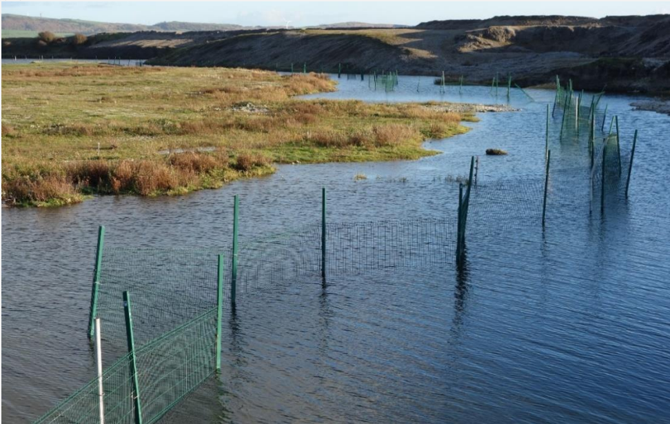
Fig. 28. Underwater fences made from V Mesh panels protecting nesting islands. (a) At Lancashire Wildlife Trust's Seaforth NR where fence posts have been driven into the substrate; (b) At Hodbarrow, where the tall panels are fixed to posts with metal plates welded to their bases which sit on the channel bed. The fence is a zig-zag shape to give it stability, and sits in water below an elevated sea bank, and so does not interrupt the view of the tern colony it protects. This photograph was taken in November, when water levels were higher than during the breeding season. Photos by Gavin Thomas.
