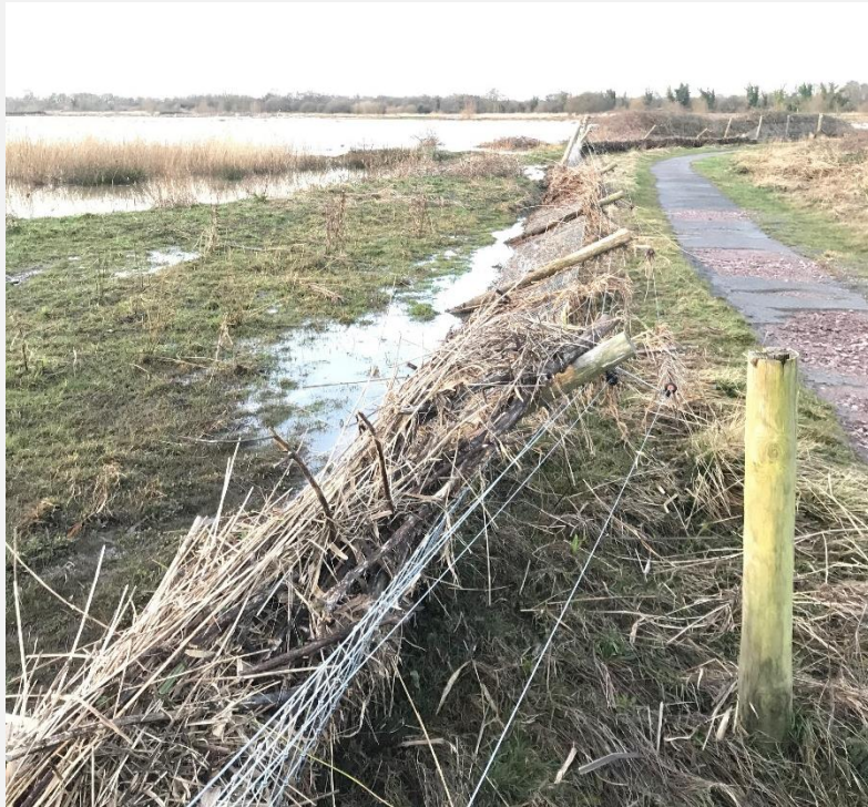
Fig. 7. A section of combination fence flattened by flood debris at Middleton Lakes in 2020. Photo by Kate Thorpe.
