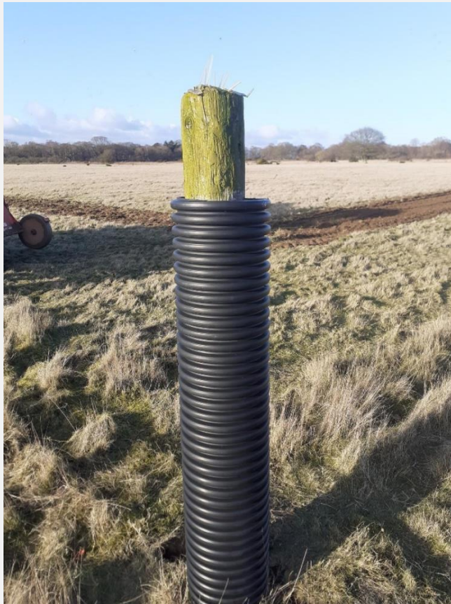
Fig. 33. A permanent, wooden corner post covered in ridged, plastic piping around which electric wires are wound when installing electric strand around Stone-curlew plots. The plastic piping is the same as that used in water management. Photo by Mel Kemp.
